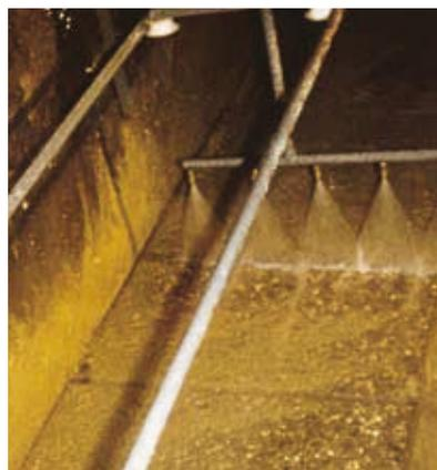
Generation of exposed aggregate concrete by fan water jets
