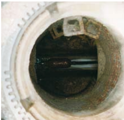
Sewer channel bottom cleaning with a Skip Jack nozzle
