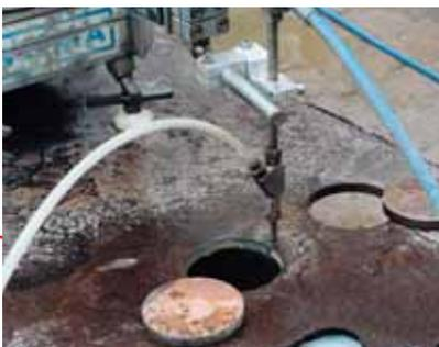
On-site cutting of openings in walls and ceilings with the 3000-bar circular abrasive cutter Eco Top Cutter.
