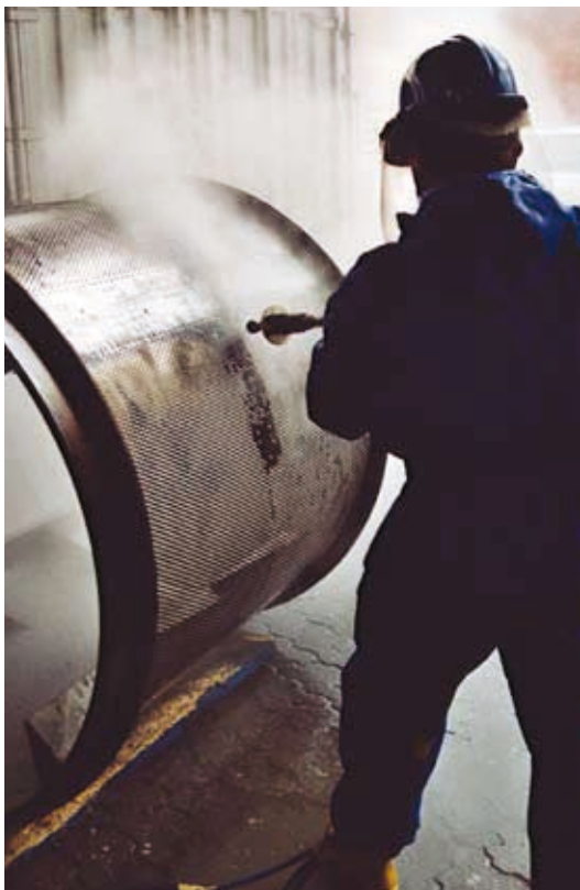
Cleaning of sieve sections with hand-held water jet tools
